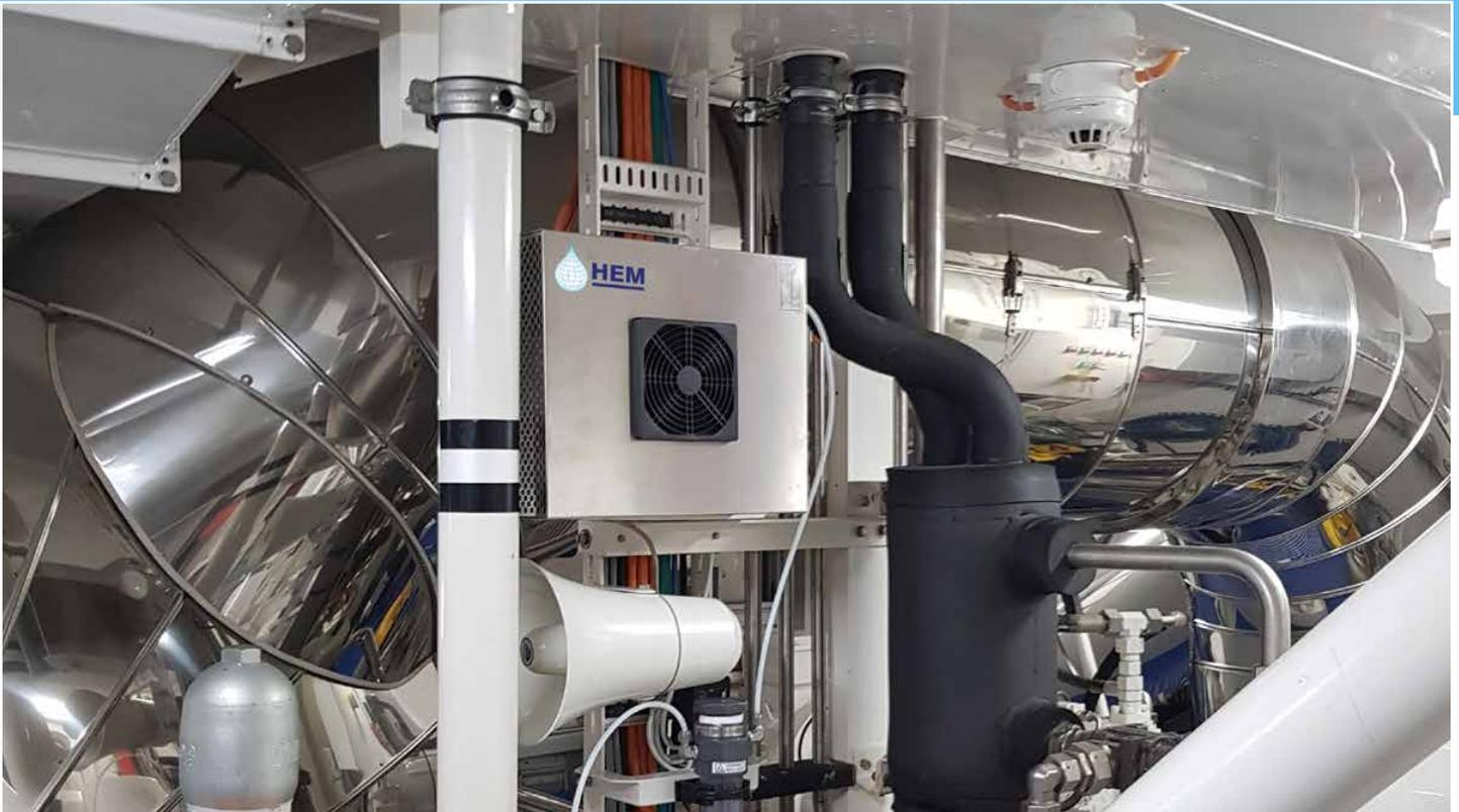
Ozone is a powerful oxidation agent used for disinfection, purification and many other applications. Ozone generators can be used for air treatment and odour removal in ventilation systems, air treatment in pump stations and sanitation after fires.
